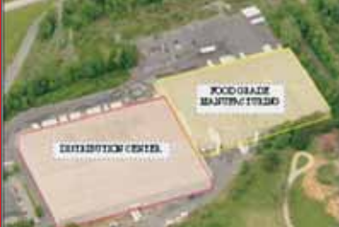
1055 Cross Road Boulevard Muhlenberg Township
