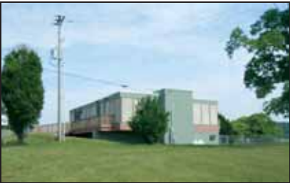
7139 Bernville Road/Route 183 Jefferson Township, Bernville
