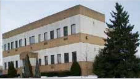
55 Raymond Street Muhlenberg Township
