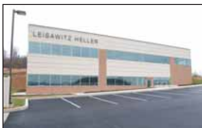
Spring Ridge 2755 Century Blvd., Wyomissing
